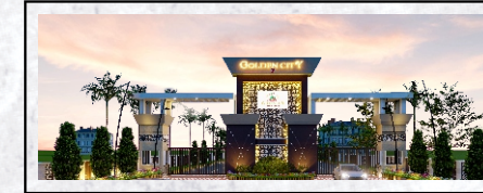
SECURED ENTRY GATE
